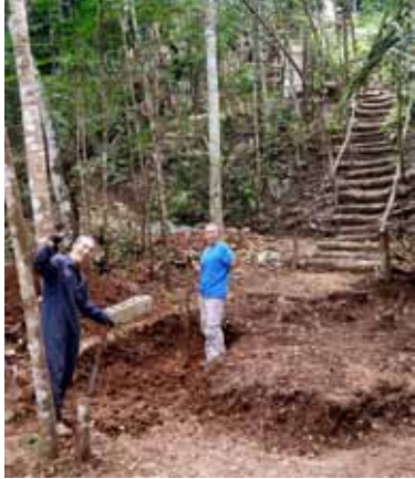
Doug and Jenny dig out the crane site
