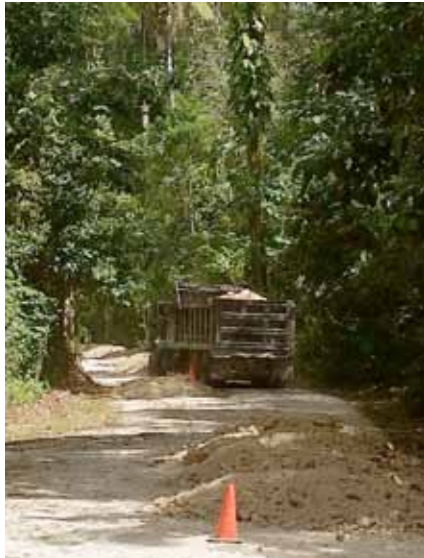
Densel's truck delivers more marl road fill
