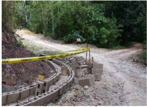
A concrete gutter will carry water around the corner
