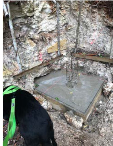
Column completed: Above
